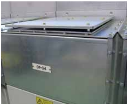
Figure 58: Example of switchgear with gas duct with top chimneys (total height of the switch-gear is 2530 mm for 12-17,5 kV up to 40 kA)
