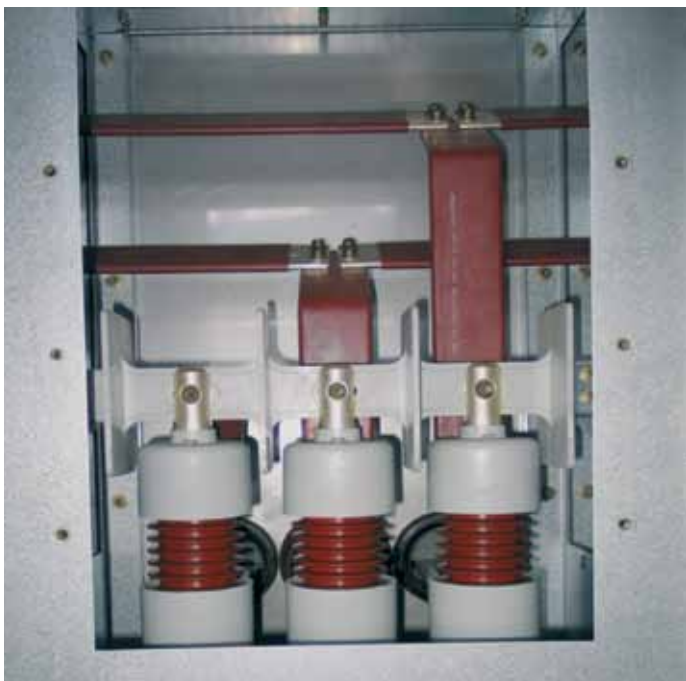
Figure 63: Closed position of busbar-disconnector
