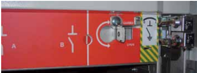
Figure 65: Front panel with operating slots of busbar-disconnector
