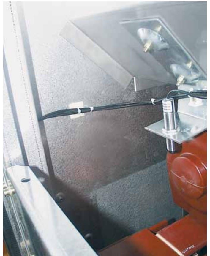
Figure 70: Example of Thermo-graphic senso in UniGear ZS1 single level
